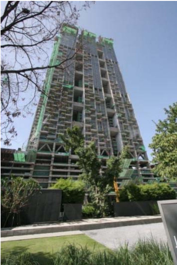
Figure 4. View of towers nearing completion
