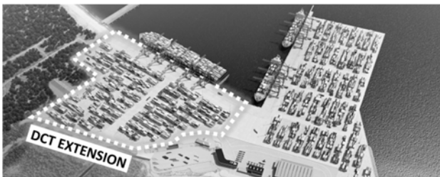
Figure 1. New berth and container stacking yards situated on the left part of the visualization (source: DCT Gdansk S.A.).
