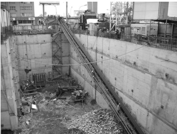
Figure 14. Ground anchors execution.
