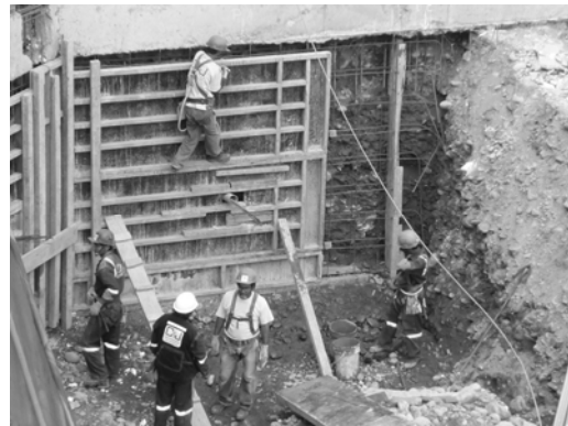
Figure 10. Formwork positioning
