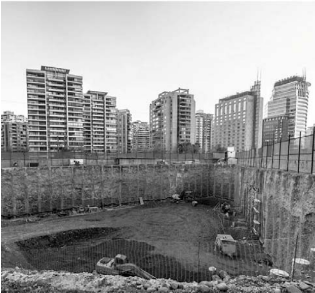
Figure 7. Parque Oriente building excavation completed.
