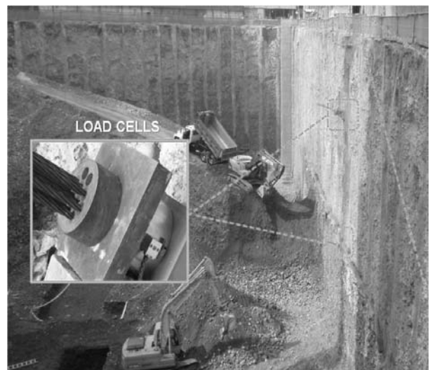
Figure 6. Load cells and instrumented pile.
