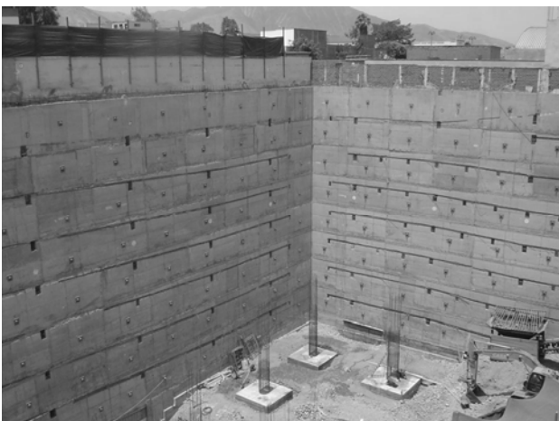
Figure 9. Anchored wall in Lima.
