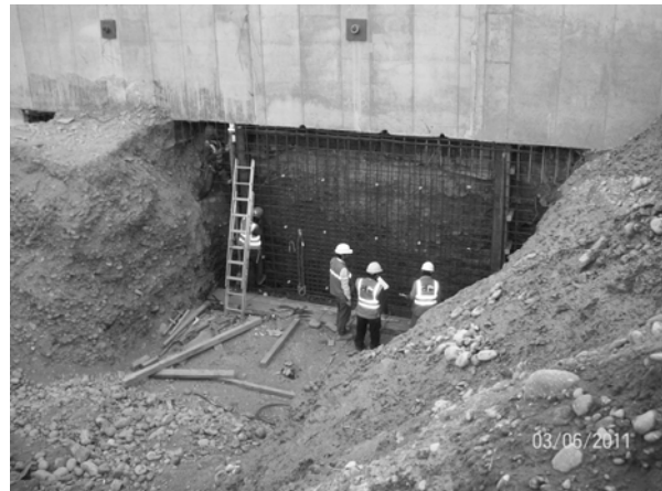
Figure 11. Steel reinforcement being place in an open panel.
