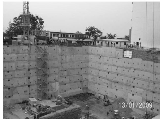
Figure 15. Republica Building with 28 m depth excavation.
