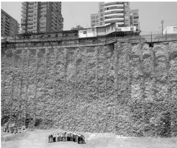
Figure 1. Deep excavation of 28 meters in Santiago.
