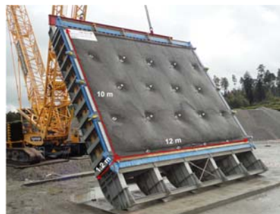
Figure 3. Test setup before the rupture of flexible facing.
