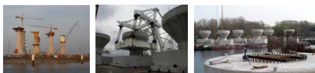
Figure 3. Offshore windfarms (a) Thornton (Belgium); (b) Nysted (Denmark); (c) Rødsand 2 (Denmark)
