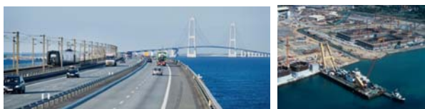
Figure 1. The Storebælt bridges, Denmark; (a) West Bridge in front & East Bridge at the back; (b) Prefab. yard for East Bridge caissons.
