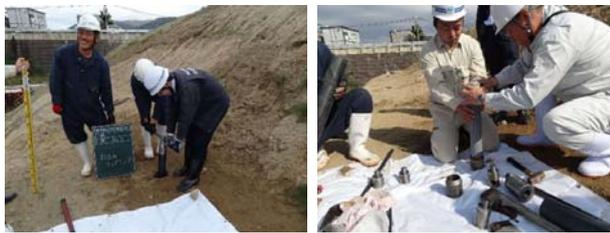
(c) Pulling out the sampler (b) Protecting the sample
