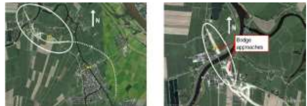
Figure 1. The new Berne bypass B212n: left: overview as per 2014; right: bridge approaches at the river Hunte
