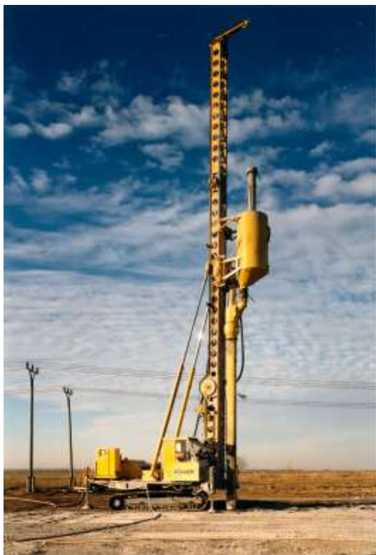
Figure 5. Installation of fly ash columns with a vibro-cat
