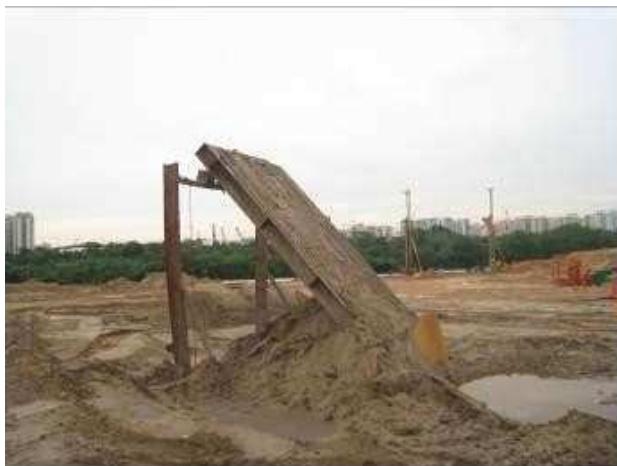
Figure 1. Mechanical sieve to segregate clay lumps and wood
