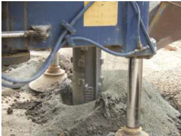
Figure 4. Installation of recycled glass sand with a vibro-cat
