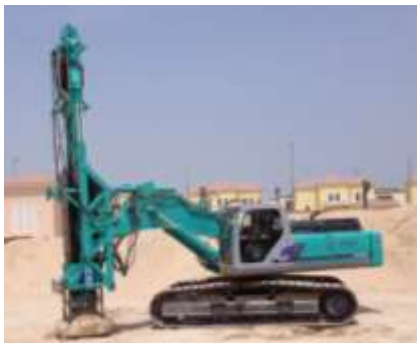
Figure 1A. Rapid Impact Compactor
