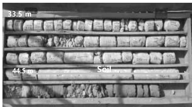
Figure 10. Concrete Core – Pile No. 1097 (Note the discontinuities and soft zones)
