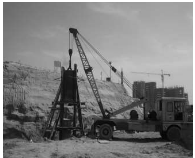
Figure 8. Dynamic Pile Load Test Setup
