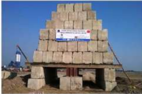
Fig. 6: Setup for Static Load Test (SLT)
