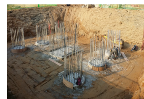
(b) Pile Head Treatment Works
