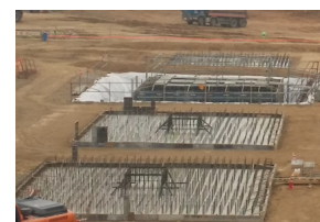
(c) Completion of Foundations for the Magnified Structure
