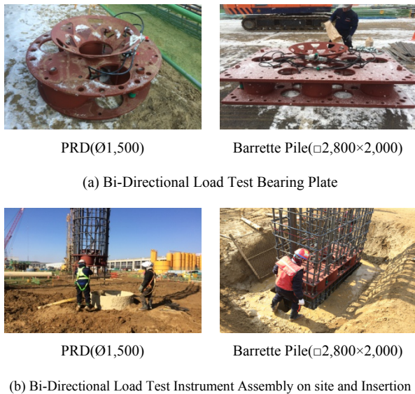
Fig.2 Sequences of the Bi-directional Load Test
