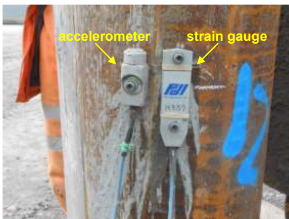
Figure 1. Accelerometer and strain gauge pair for measuring transferred energy on a DCIS pile tube
