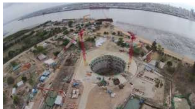
Figure 1. Southern shaft before installation of anchorage block inside
