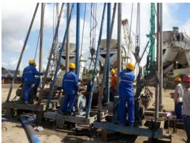
Figure 4. Concreting one panel by tremie method
