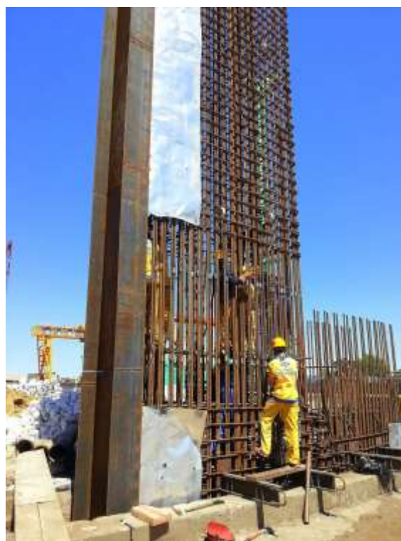
Figure 3. Installation of reinforcement cage with special steel joint
