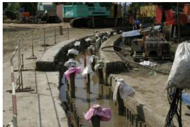
Figure 6. CSL – tubes at head of diaphragm walls for testing
