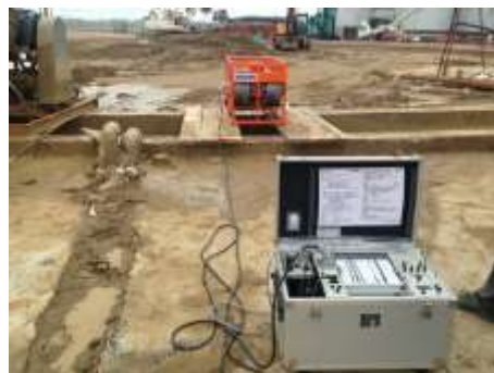
Figure 2. Testing of the panels for verticality and shape after execution
