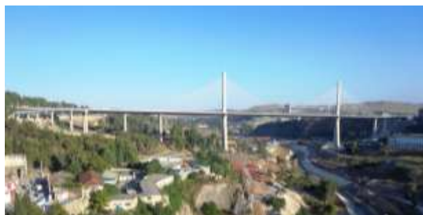
Figure 5. View of completed Transhumel Viaduct, Constantine, Algeria
