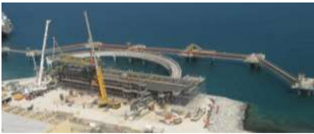
Figure 7. Ruwais Sulphur Expansion project. Quadrant beam, mooring and breasting dolphins.
