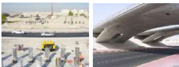
Figure 4. Wali Al Ahed flyover; (a) bored piles; (b) completed structure
