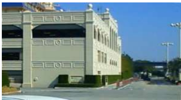
Photo 1. View of ground around the building (March 13, 2011)
