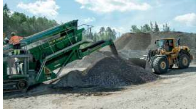
Figure 1. High quality CCA crushed to stockpile
