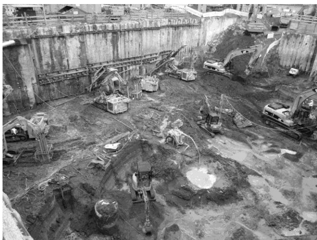
Figure 8. Anchor installation during excavation.
