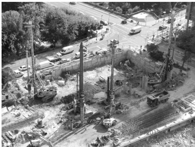
Figure 7. Construction of the bored pile wall.
