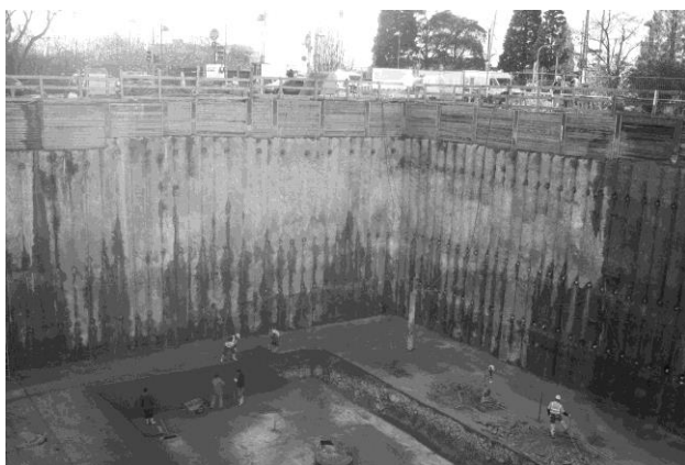
Figure 9. Construction of the blinding concrete layer.
