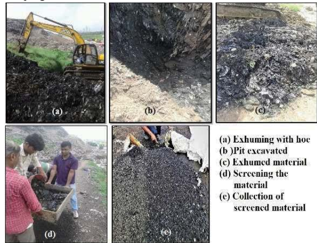
Figure 1. Excavating and screened MSW from Pirana
