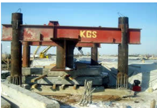
Figure 4. Test by static loadings.
