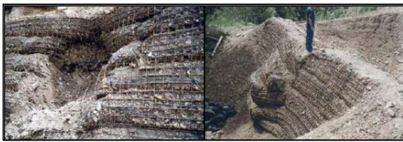
Fig. 1. Embankment impacted without reaching collapse
