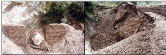
Fig. 2. Collapsed impacted embankment
