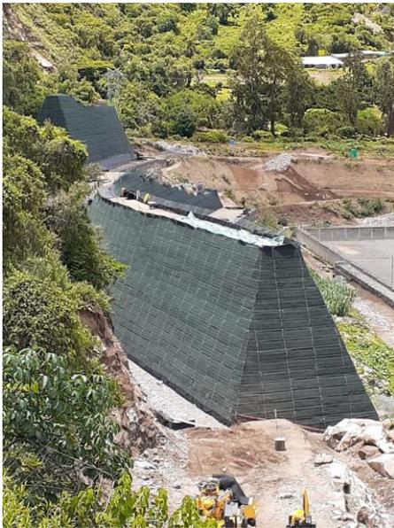
Figure 11. Execution of static barrier with soil reinforced wall
