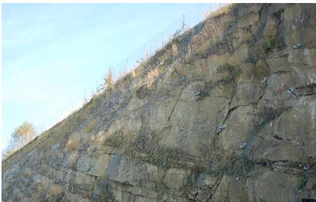
Figure 4. Option 1. Rockfall protection by the Geobrugg TECCO mesh and Ischebeck TITAN rock bolts, Poland.
