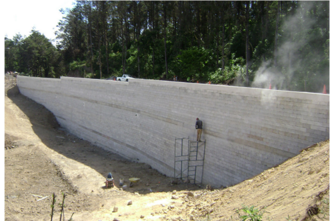
Figure 11. Final state of the wall (courtesy GSS Titan)
