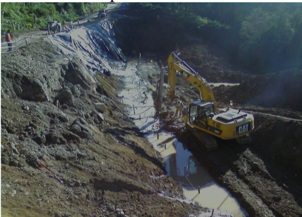
Figure 10. Micropile installation (courtesy GSS Titan)
