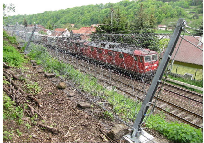
Figure 5. Option 2. Rockfall barriers along railway tracks, founded on TITAN micropiles, Germany
