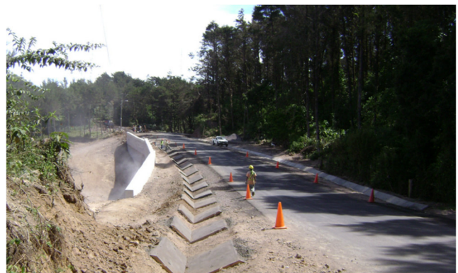
Figure 12. Repaired route 228 Colpachi - Cartago (courtesy GSS Titan)
