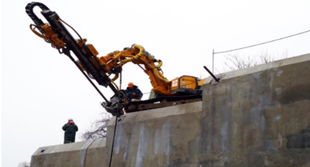
Figure 7. Installation of TITAN anchor piles on top of a retaining wall.
