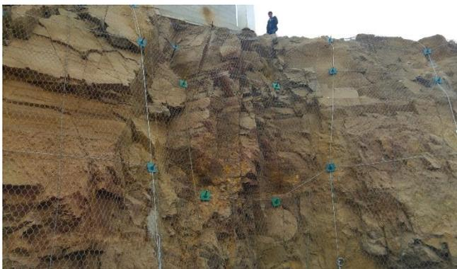
Picture N° 07: Slope Reinforcement
