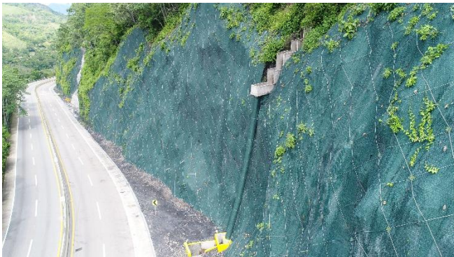
Figure 14. Steel and PVC coated mesh.
