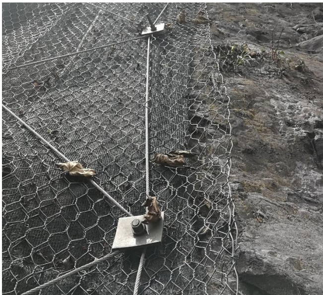
Figure 10. 15cm x 15cm steel plate and hexagonal nut
