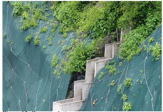
Figure 13. Concrete drainage system.
