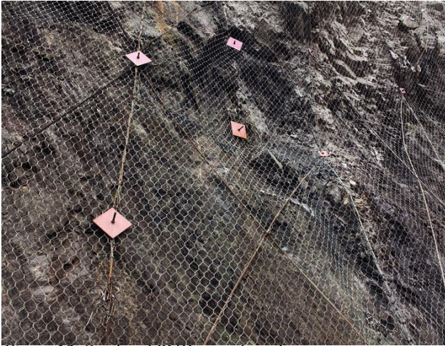
Figure 13. Steel and PVC coated mesh
