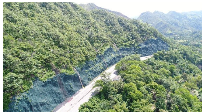
Figure 8. General view of the slope intervened by green system
