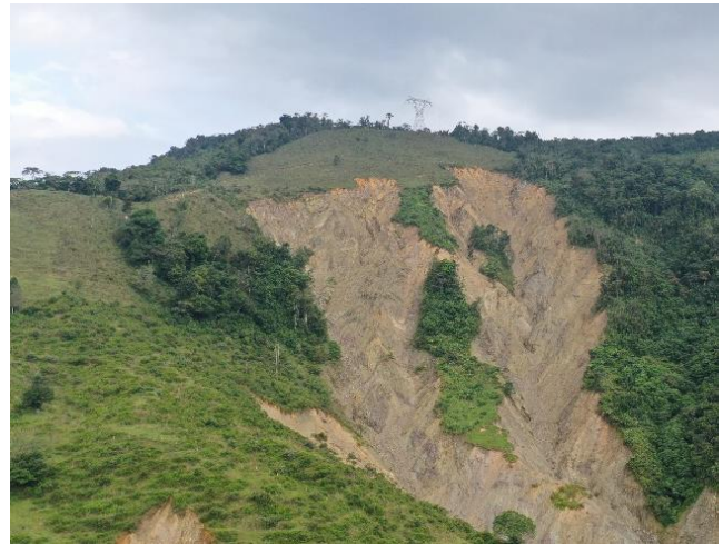
Figure 7. Advancement of the slope degradation process near a power tower.
