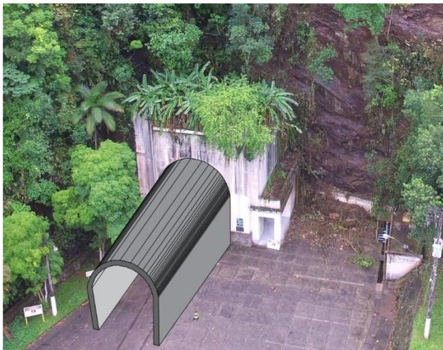
Figure 5 - False tunnel, initially considered as a solution
