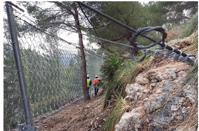
Figure 9. New dynamic barrier on Formentor rockfall area (April 2017 image)
