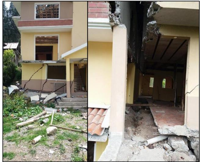
Figure 1. Examples of building damage in Cuenca induced by landslides.
