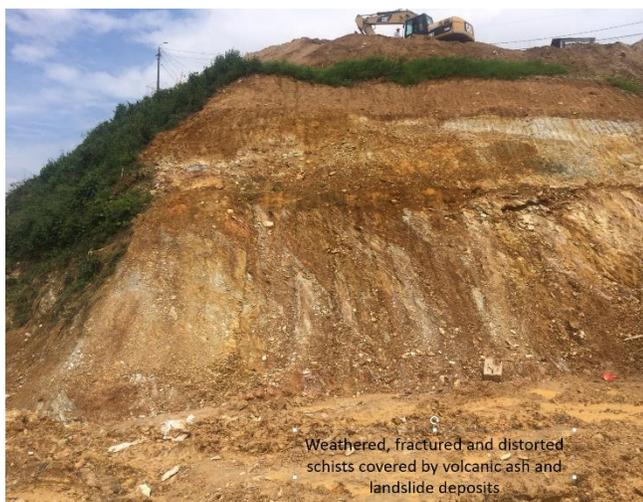
Figure 6 - Excavation slope in fractured schists and surface cover to the east of the fault zone.
