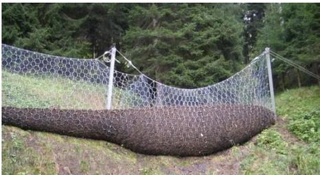
Figure 2. Rockfall barrier loaded with a shallow landslide.
