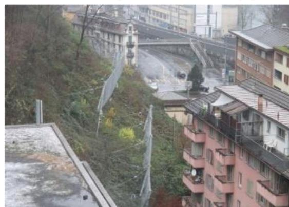
Figure 13. Shallow landslide barrier in Luzern Güttsch Switzerland as direct property protection.
