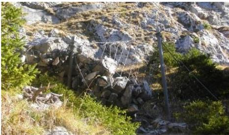
Figure 1. Snow net barrier loaded with rockfall
