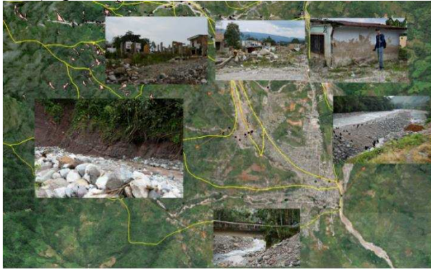
Figure 3. Evidence of destruction caused by the debris flow moving along Taruca creek valley, in Mocoa.
