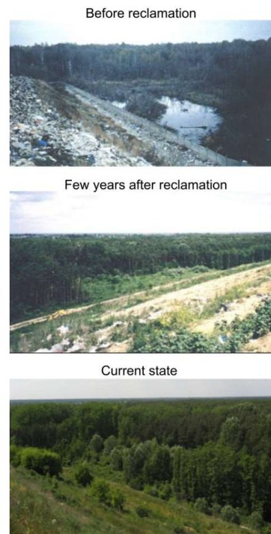
Fig. 5. Effects of biological reclamation of the Lubna landfill (view on the northern slope before and after reclamation works).
