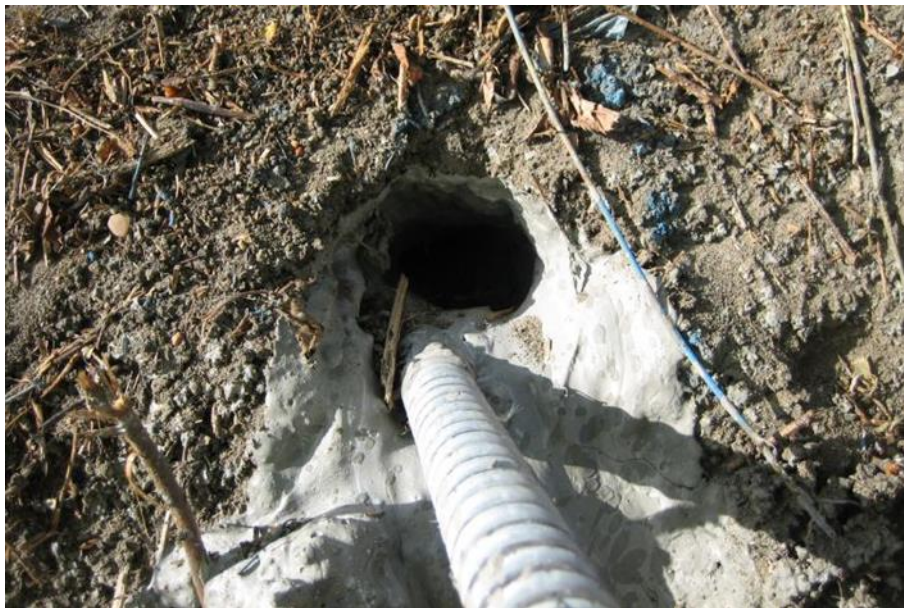
Figure 4: Self-drilled soil nail lying on the base of the borehole due to failure to use centralisers. This reduces the grout cover for corrosion protection and potentially reduces the bond strength.
