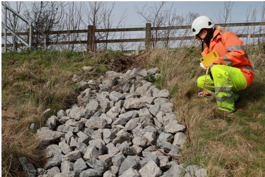
Figure 3: Settlement of large-sized drainage media at the head of a counterfort drain.
