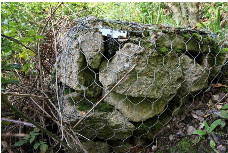
Figure 2: Oversize concrete fill leading to large voids within the gabion baskets. The oversize fill also means that the gabions have been unable to be properly sealed along the top, instead they are secured at pinch points where the fill allows.
