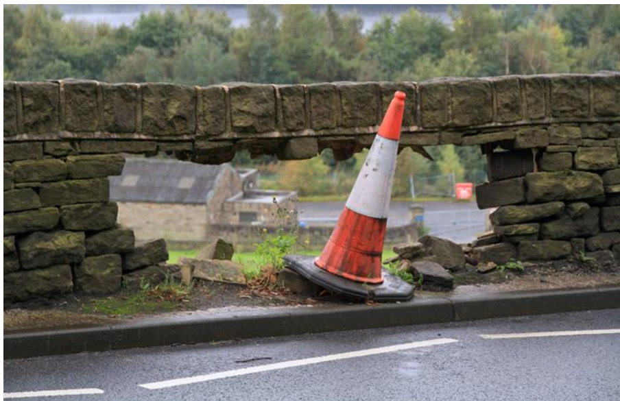
Figure 1: Upper free-standing part of a dry-stone retaining wall (mortared coping) showing the effects of vehicle impact. The wall below the carriageway retains a height of between 2m and 3m below the road.
