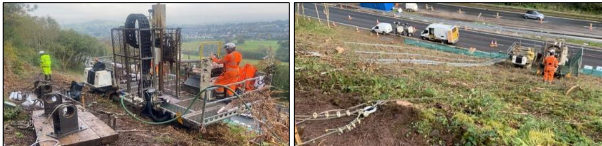
Figure 4: On-slope ground investigation, showing crest anchor system.
