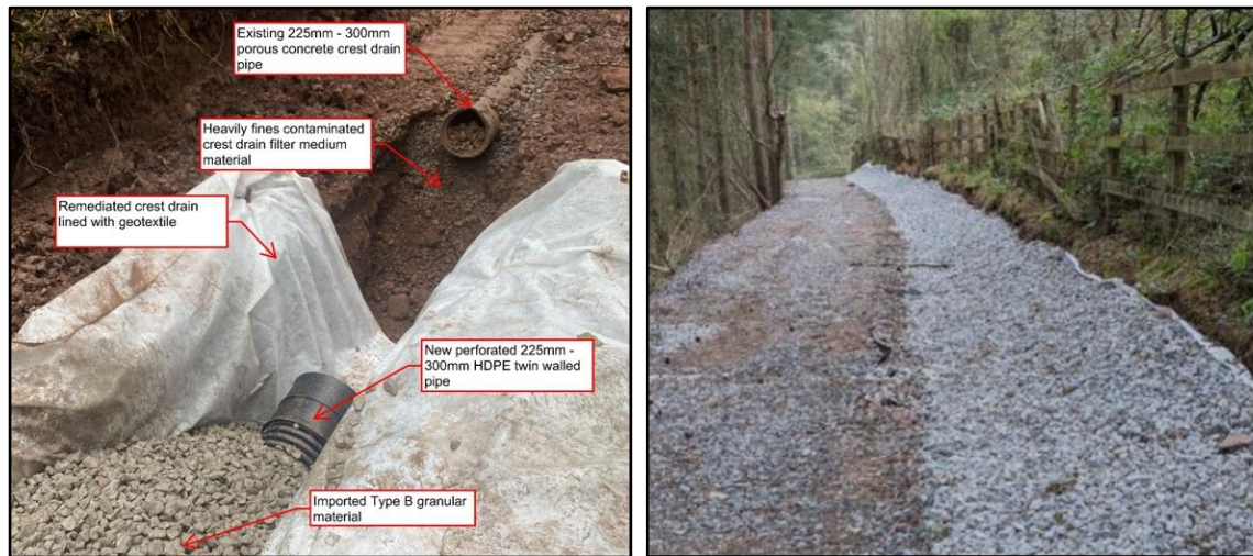
Figure 7: Renewal of the crest drain. Left: replacement of pipework and filter media. Right: completed works.
