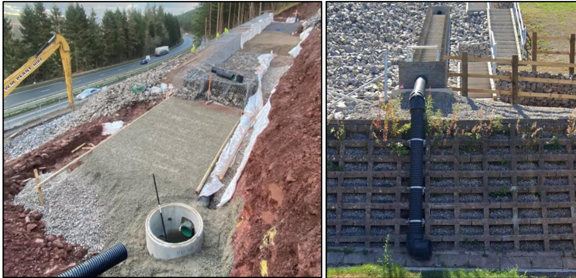
Figure 8: Left: gabion wall and associated drainage construction, right: cascade and over-wall drainage pipe.
