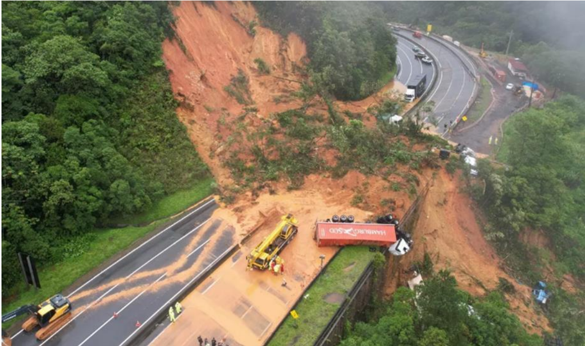
Figure 1: Recent landslide dated 28 November 2022 in Brazil. Image from CBMSL via MetSul.com.
