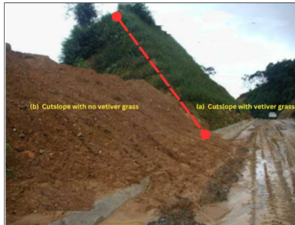
Figure 8. Ho Chi Minh Road slope (a) Before, (b) After being planted for protection with vetiver grass (Tran et al., 2014)).
