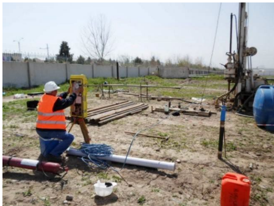
Figure 4. Conducting Pressuremeter test at the same location
