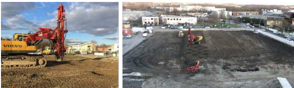
Figure 4. Rapid impact compaction (R.I.C.) for brownfields.
