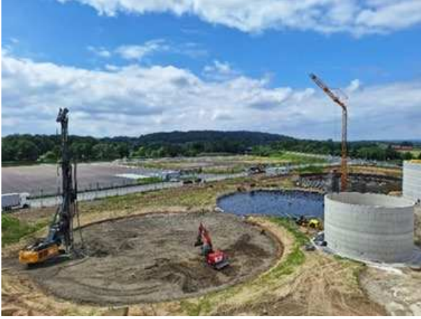
Figure 5. CMC execution for the tank foundation.
