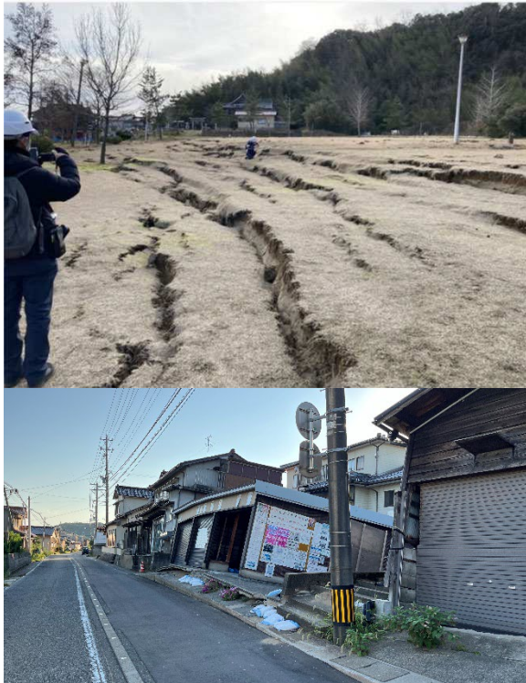
Figure 2. Damages from liquefaction in Uchinada Town
