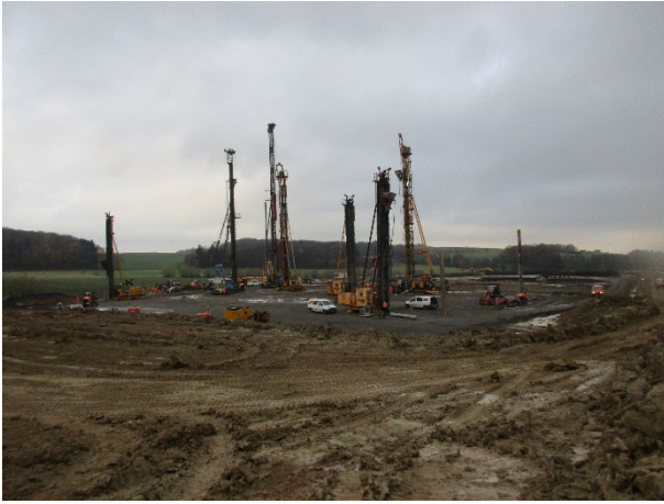
Figure 11. Deep foundation rigs.
