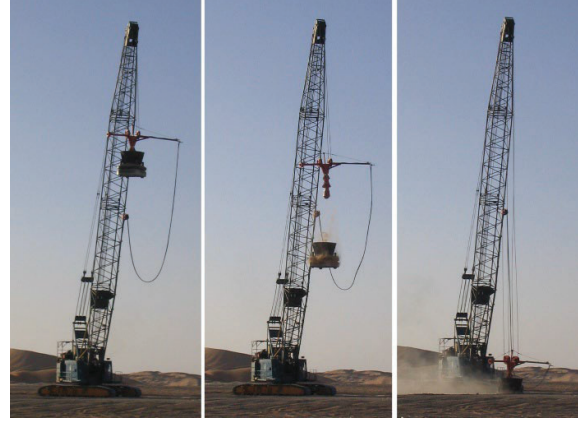
Figure 6. Application of DC using 35-t poulder (Hamidi et al. 2010a)
