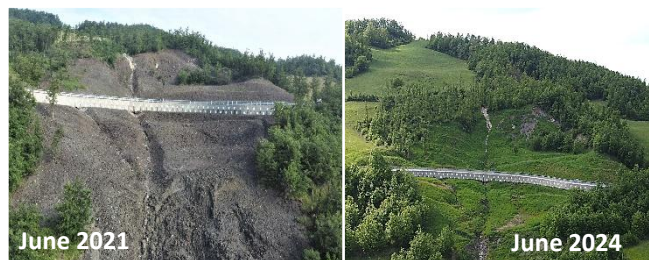
Figure 1. The Castiglione dei Pepoli site, as observed in June 2021, exhibited no erosion control measures and was affected by severe hydrogeological instability. By June 2024 successful Nature-based solutions were implemented
