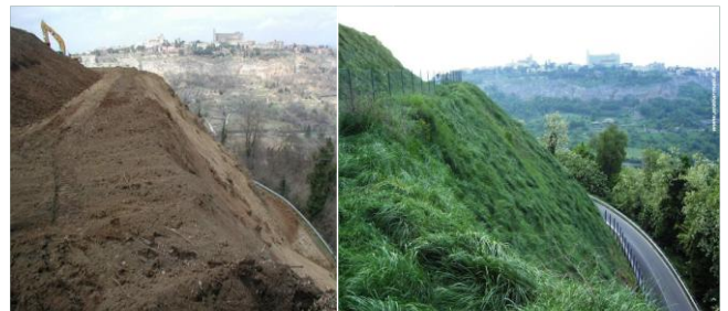
Figure 4. Field experiments conducted by the Department of Geology at the University of Perugia demonstrate a reduction in soil loss from 1008.84 to 0.06 ton/hect/year, three years after the intervention
