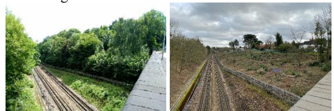
Figure 4. Chigwell Cutting Vegetation Clearance Before and After
