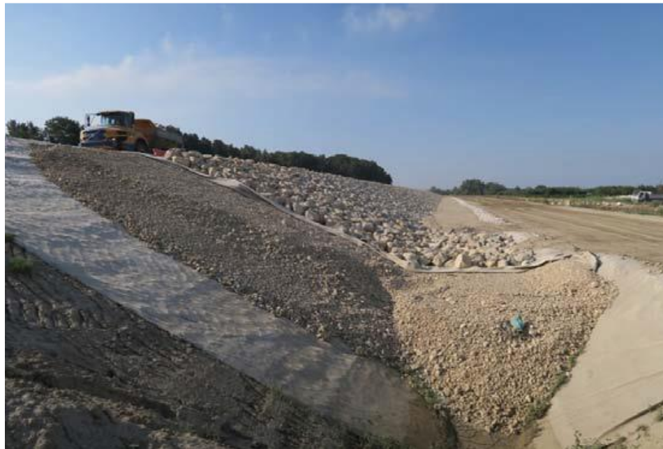
Figure 2. Filters on downstream slope and in drainage trench, flood levees, Rhone Delta Project (courtesy Thibaut Mallet, Symadrem, France).
