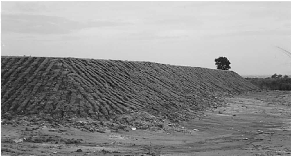
Fig. 21 – Reinforced embankment
