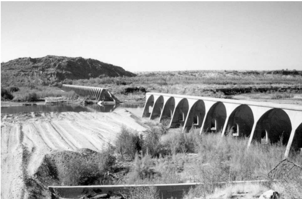
Figure 7. Failed portion of the Gillespie Dam just upstream from the US-80 Bridge
