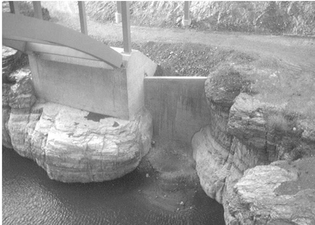
Figure 11. Completed repair of scour hole
