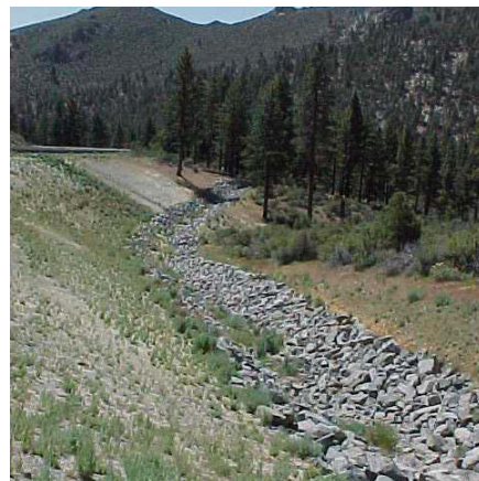
Figure 4. Channel lined with rip rap
