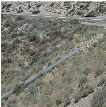
Figure 3. Culvert with a pipe slope drain
