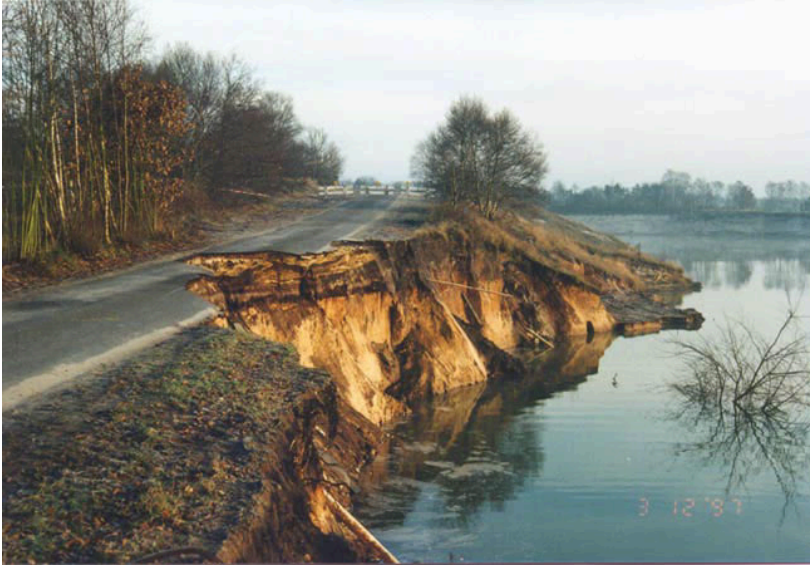
Figure 21 – Bank collapse due to scouring
