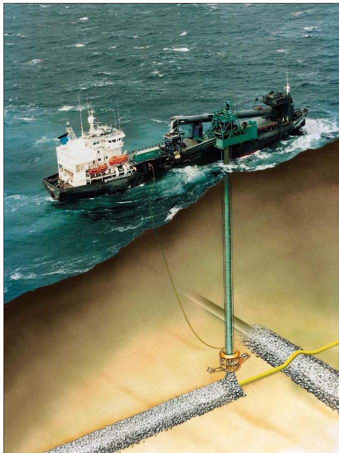
Fig. 5 – Flexible Fall Pipe Vessel “ Trollnes ”
